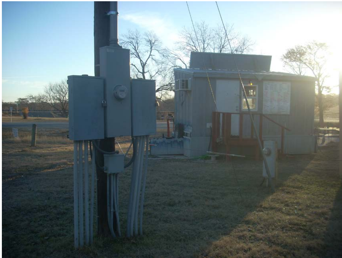
Figure #8 – Existing Electrical Service Panels at Park Entrance
